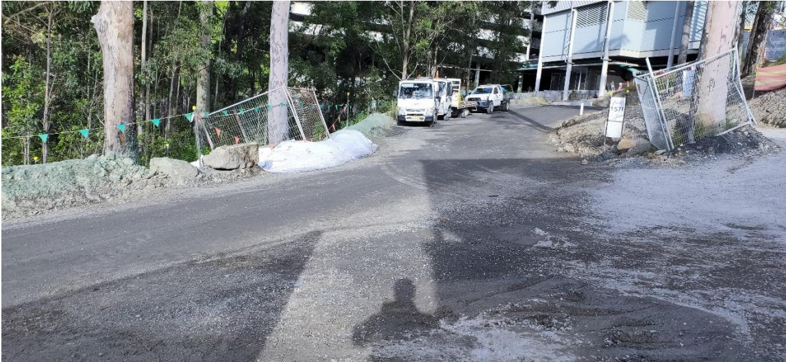
Photograph 4 – Temporary access road sealed
