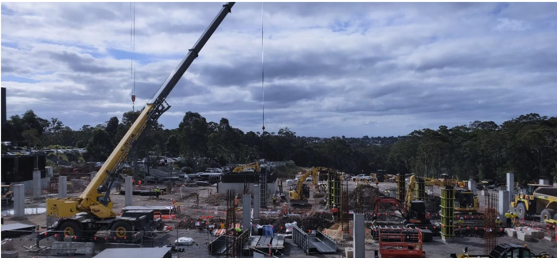
Photograph 5 – ABS looking North
