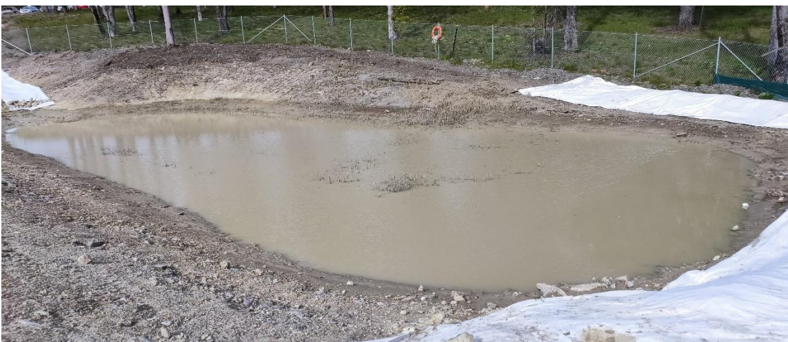
Photograph 6 – Basin on east-west access road
