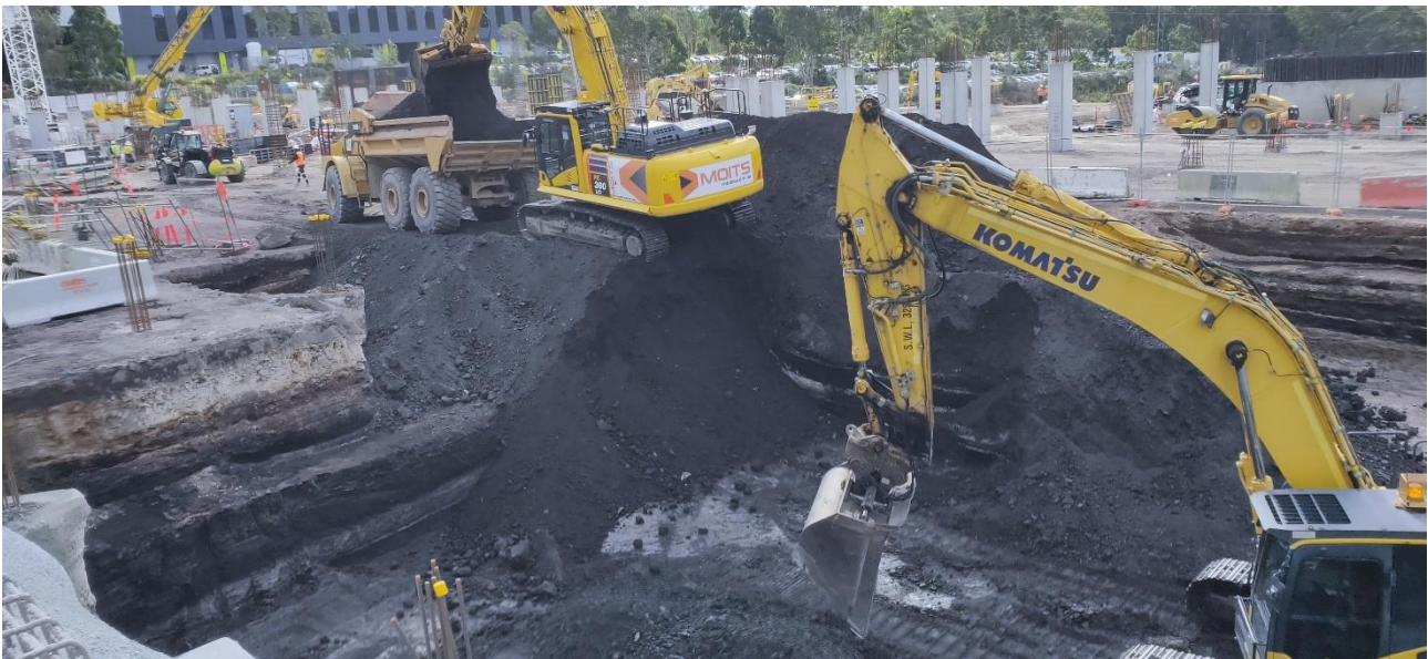
Photograph 8 – Bulk excavation ASB looking north-west
