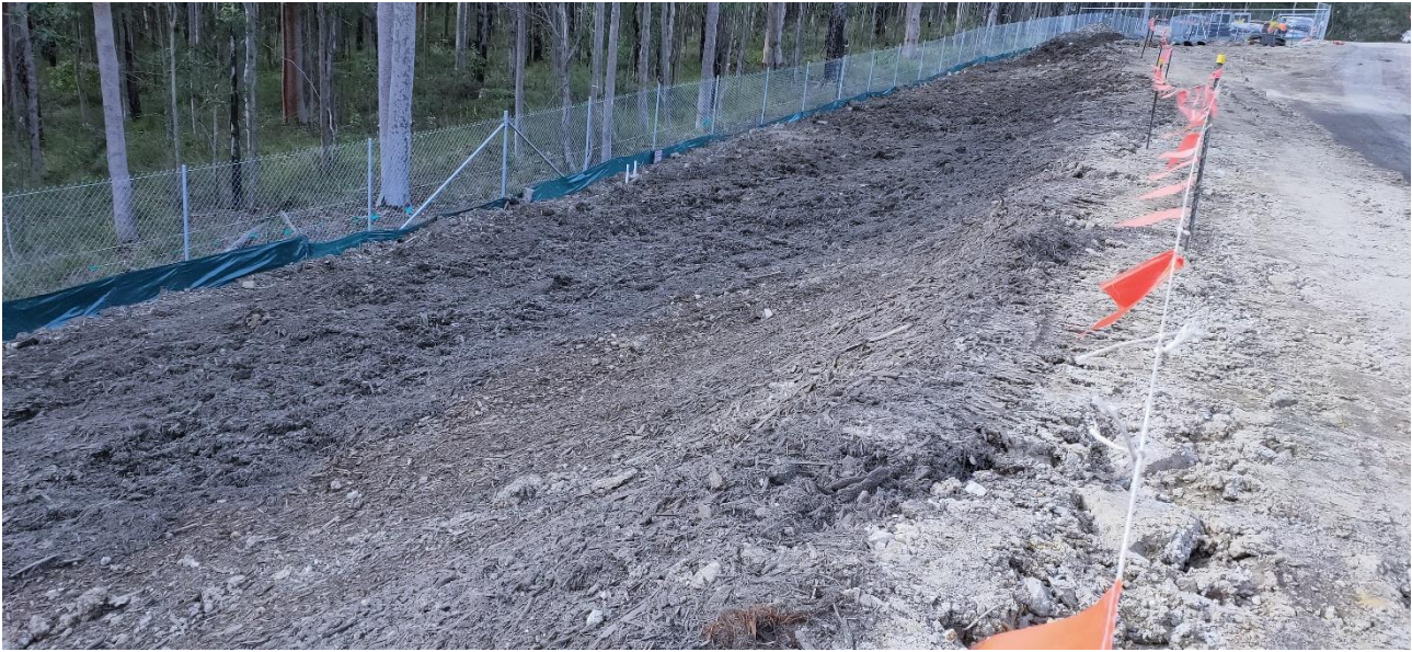
Photograph 7 – Batter slope treatment east west access road 2
