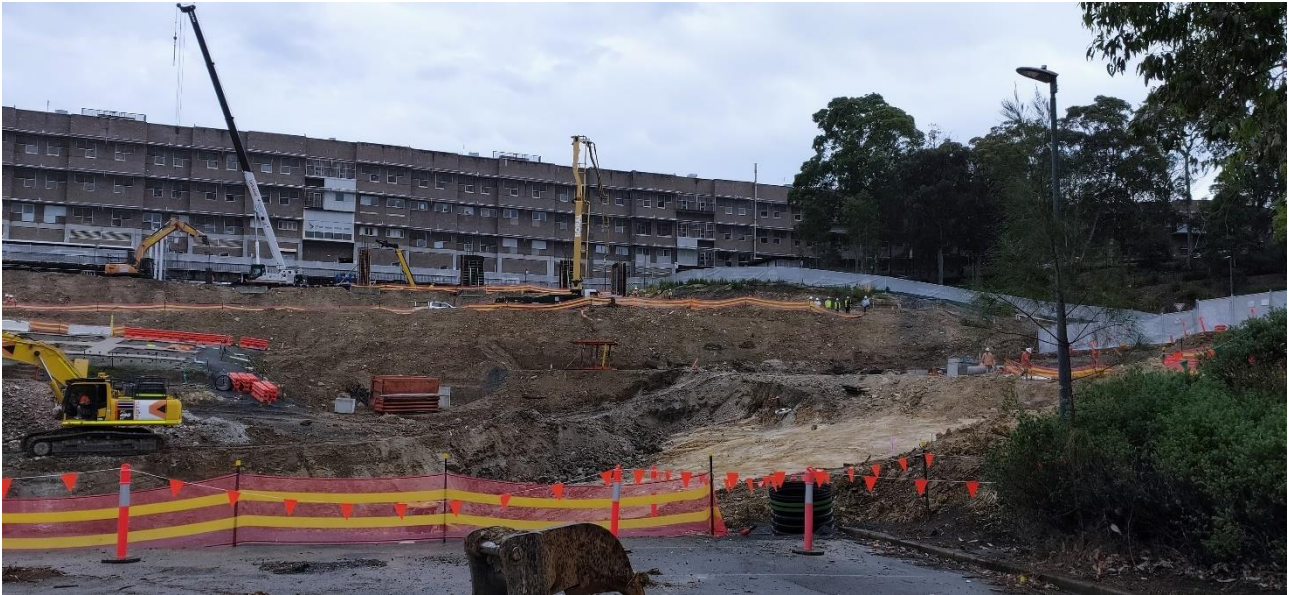
Photograph 2 – Site conditions looking south
