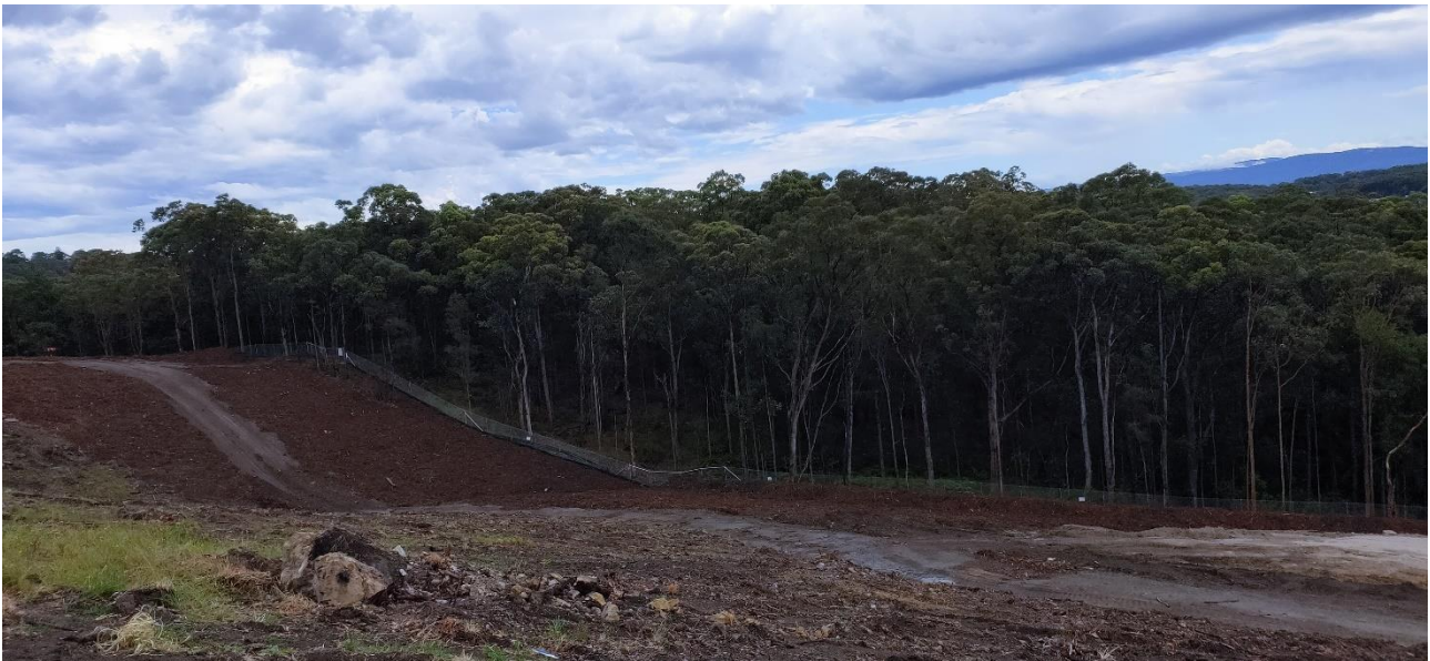
Photograph 3 – Western access road clearing completed and stabilised
