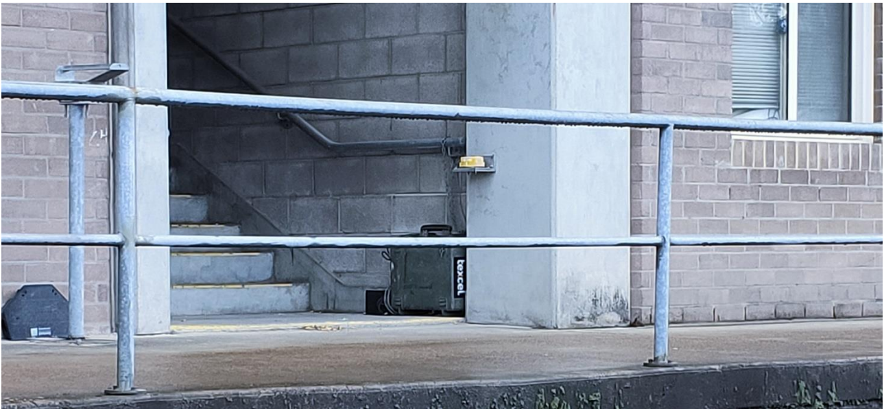
Photograph 5 – Vibration monitor in place on John Hunter Hospital building
