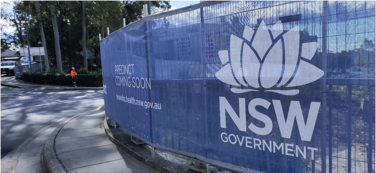
Photograph 6 – Site screening in place Kookaburra Circuit
