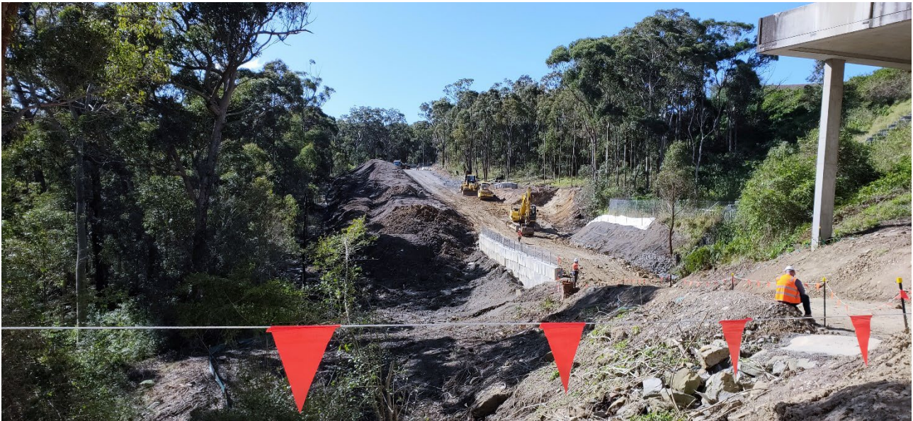
Photograph 2 – Site conditions looking east
