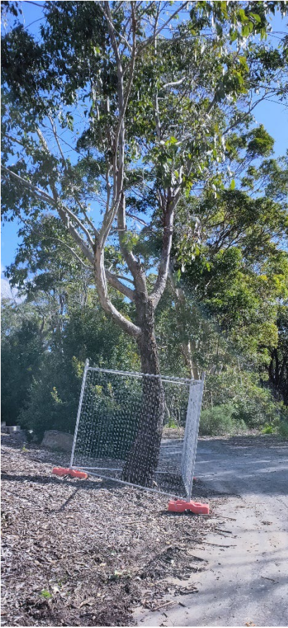
Photograph 13 – Tree protection around retained tree
