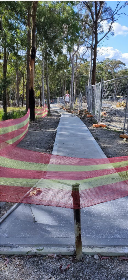
Photograph 14 – New pedestrian route from carpark nearing completion
