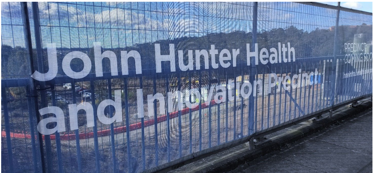
Photograph 11 – Site screening installed
